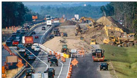
Maine Turnpike Widening and Modernization Project, Biddeford/Scarborough, Maine
