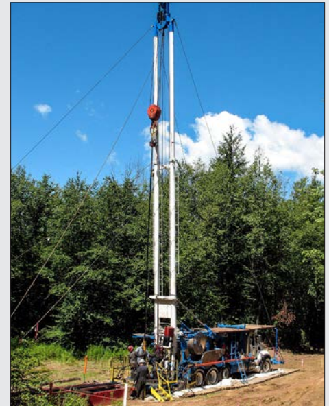
Oil well plugged with a double-pole service rig
