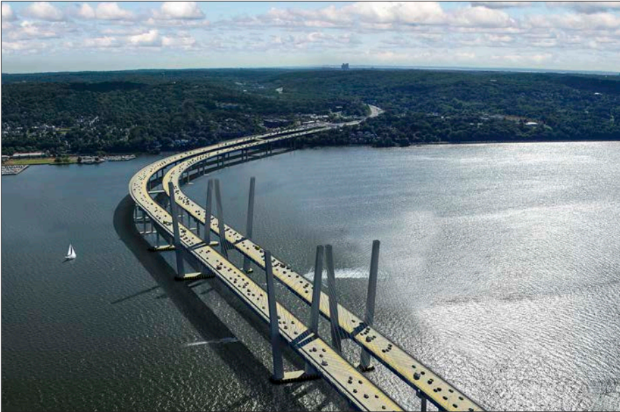
The New NY Bridge, Tarrytown, NY. courtesy of New York State Thruway Authority
